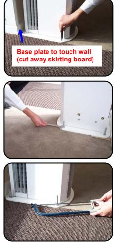
Remove only one M10 nut and refit and resecure bolt with a stainless steel M10 dome nut supplied. Repeat for each of the other three projecting bolts one at a time.
